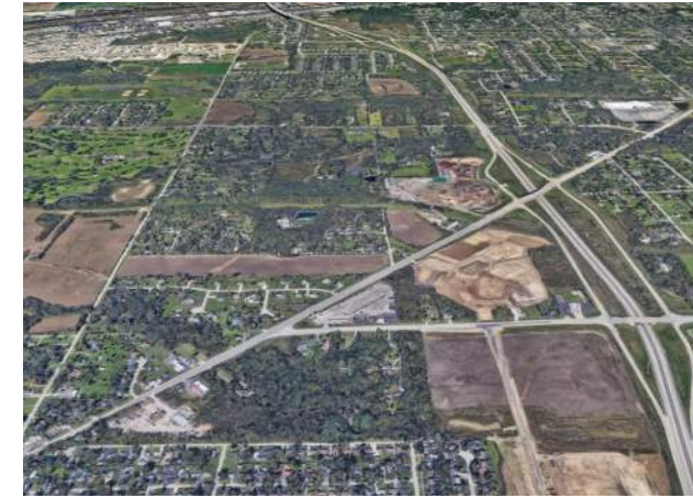
Route 171 interchange on I-355
